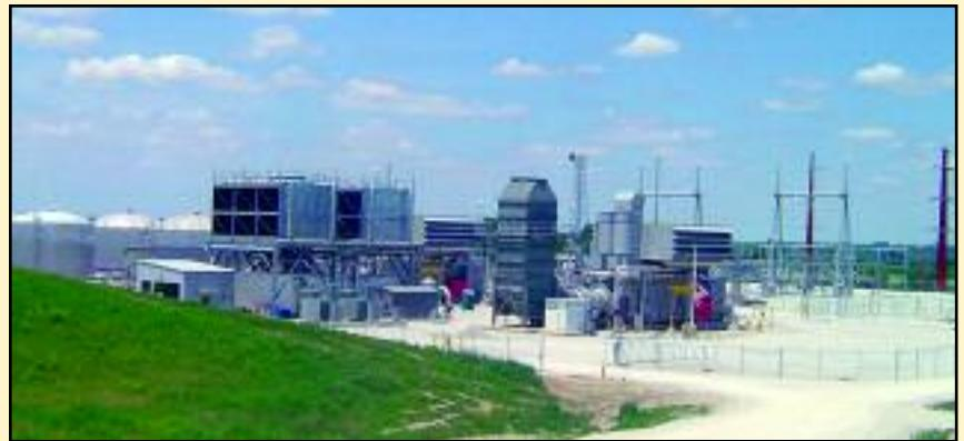
An inlet chilling system allows the facility to operate at peak output and efficiency year round. Photo courtesy of TAS, Ltd.
